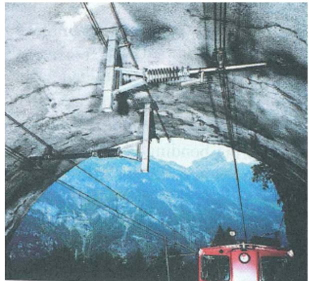
Figure 1: Applications of Composite insulators in European Railways network – Lotschberg tunnel [8]
