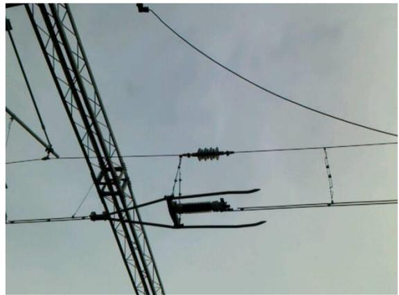
Figure 4: Use of HV insulators for Railway applications; example: 2
