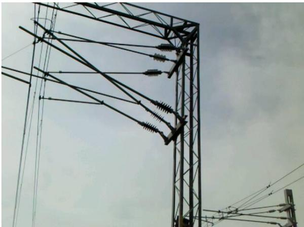
Figure 3: Use of HV insulators for Railway applications; example: 1
