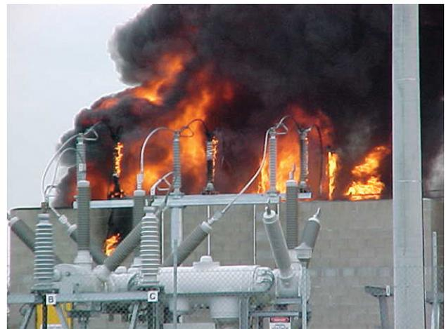
Figure 1: A 110-kV OIP bushing failure caused this 80-MVA transformer fire [5]
