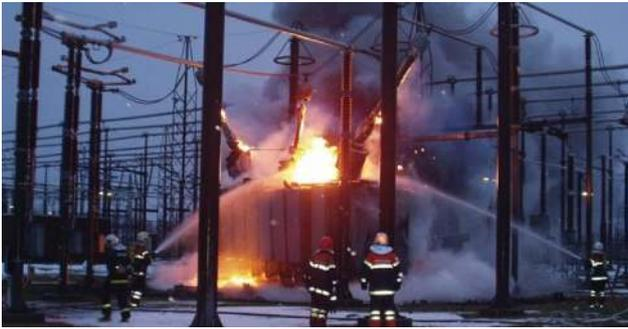
Figure 2: An OIP bushing failure on the 400-kV, 100-MVAR reactor caused this reactor fire [5]
