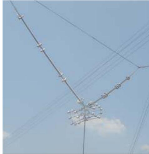
**1,200-kilovolt insulators from Deccan in grid operation (photo on left) and during application tests (right).**
